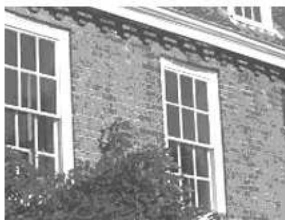
Photo. 7. Flemish bond brickwork, and another fine denticulated cornice, Millgate.
