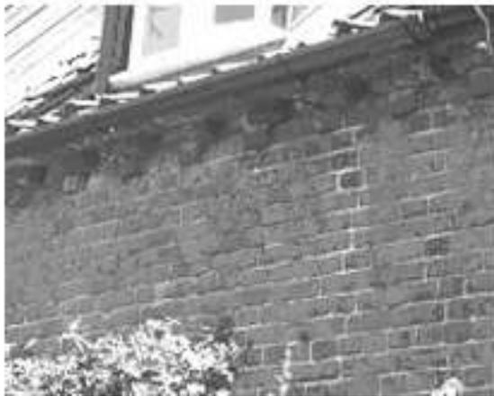
Photo. 6. English bond brickwork, and a denticulated cornice, Millgate.
