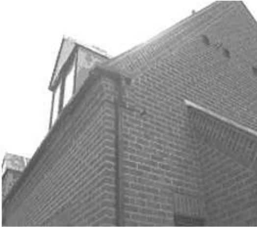
Photo 8. Stretcher bond brickwork, sloping brickwork on the gable and brick cornice on a modern building, Mill Row.
