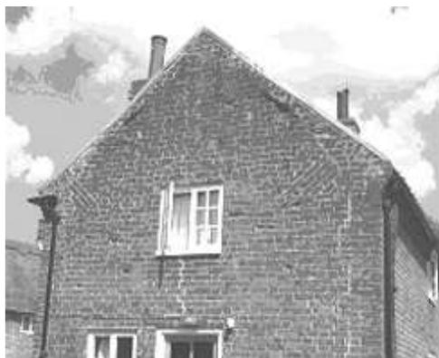
Photo. 4. This house in Silvergate shows how bricks can be laid at angle to strengthen the gable parapet, called ‘tumbling’.
