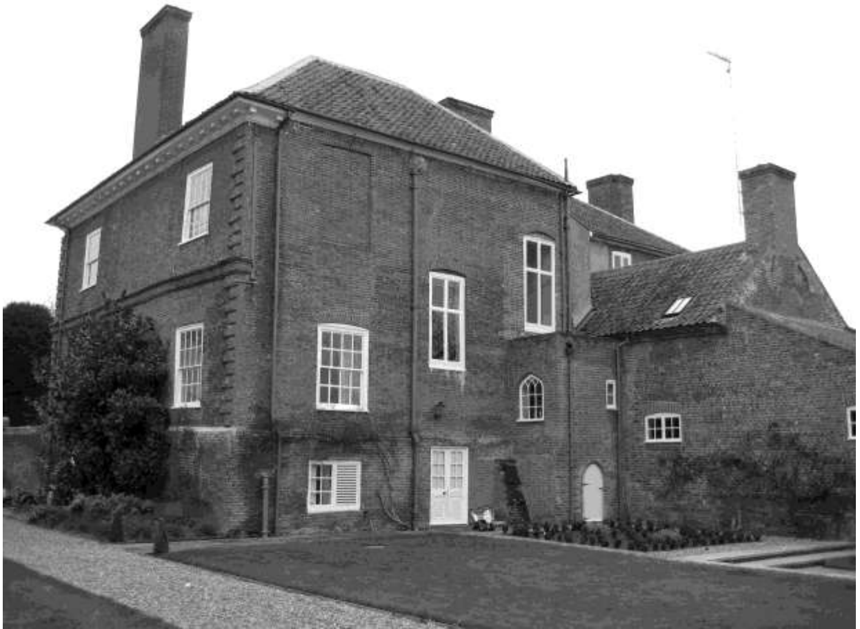
The central old mullioned window on the east facade
