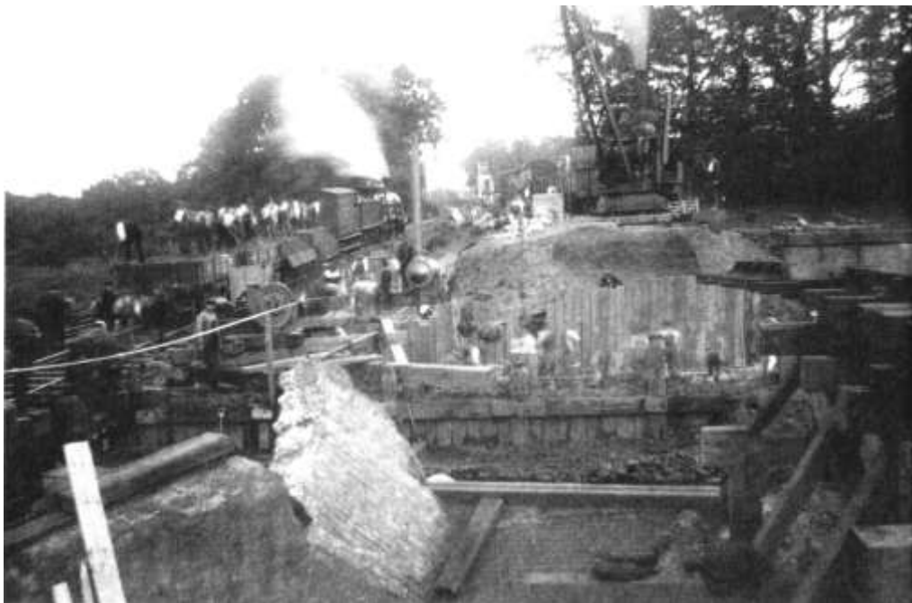
Repairing Blackwater Bridge
