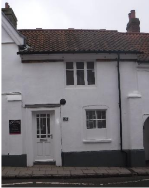
35 Market Place doorway restored in place of ATM
