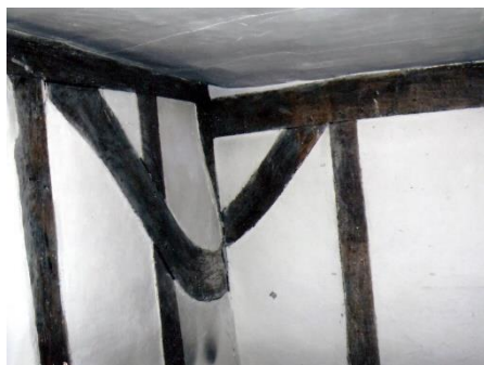
Corner SW gable First floor
