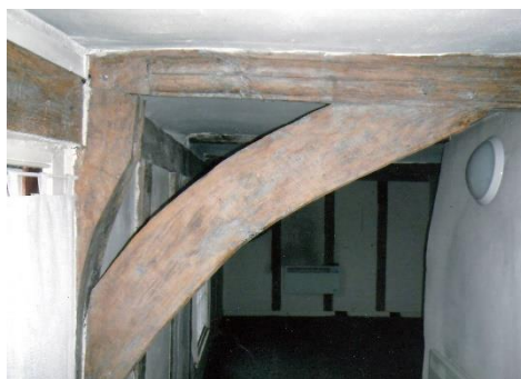
First floor looking north: main brace and chimney stack
