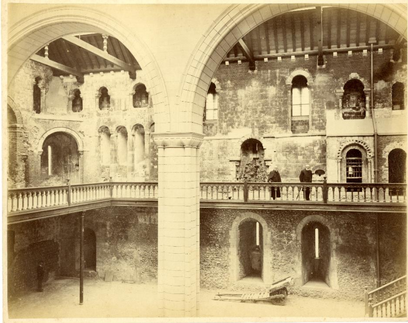
Photograph of South-east corner of the Keep during the conversion to a museum, 1890-2 (Norfolk Museum Service)
