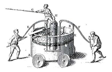
Is this what Aylsham's fire engine looked like? The drawing is a contemporary illustration of a fire engine, taken from "The Motion of fluids, natural and artificial, in particular that of air and water" by M. Clare. 2nd. ed 1737
